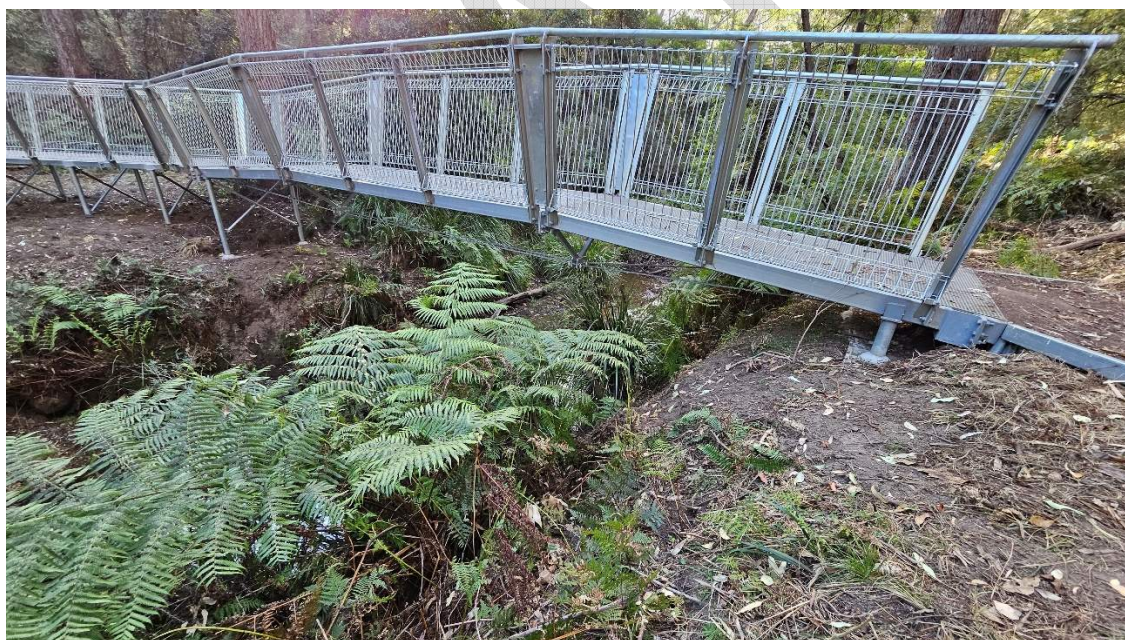
Example of platform with both footing and clear span sections – Narooma NSW
